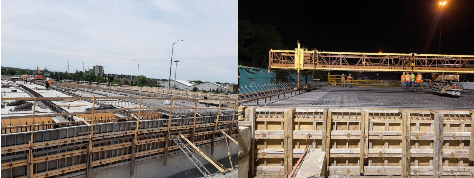
Figure 1: Typical Concrete Deck Pour Setup
